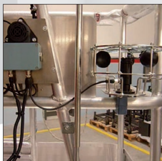
Wind speed control device, with alarm.
